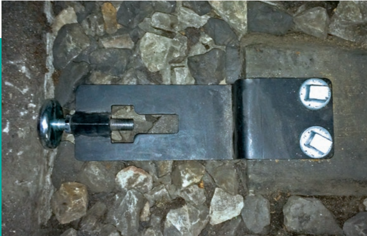
Assembly on wooden sleeper – with drilling
